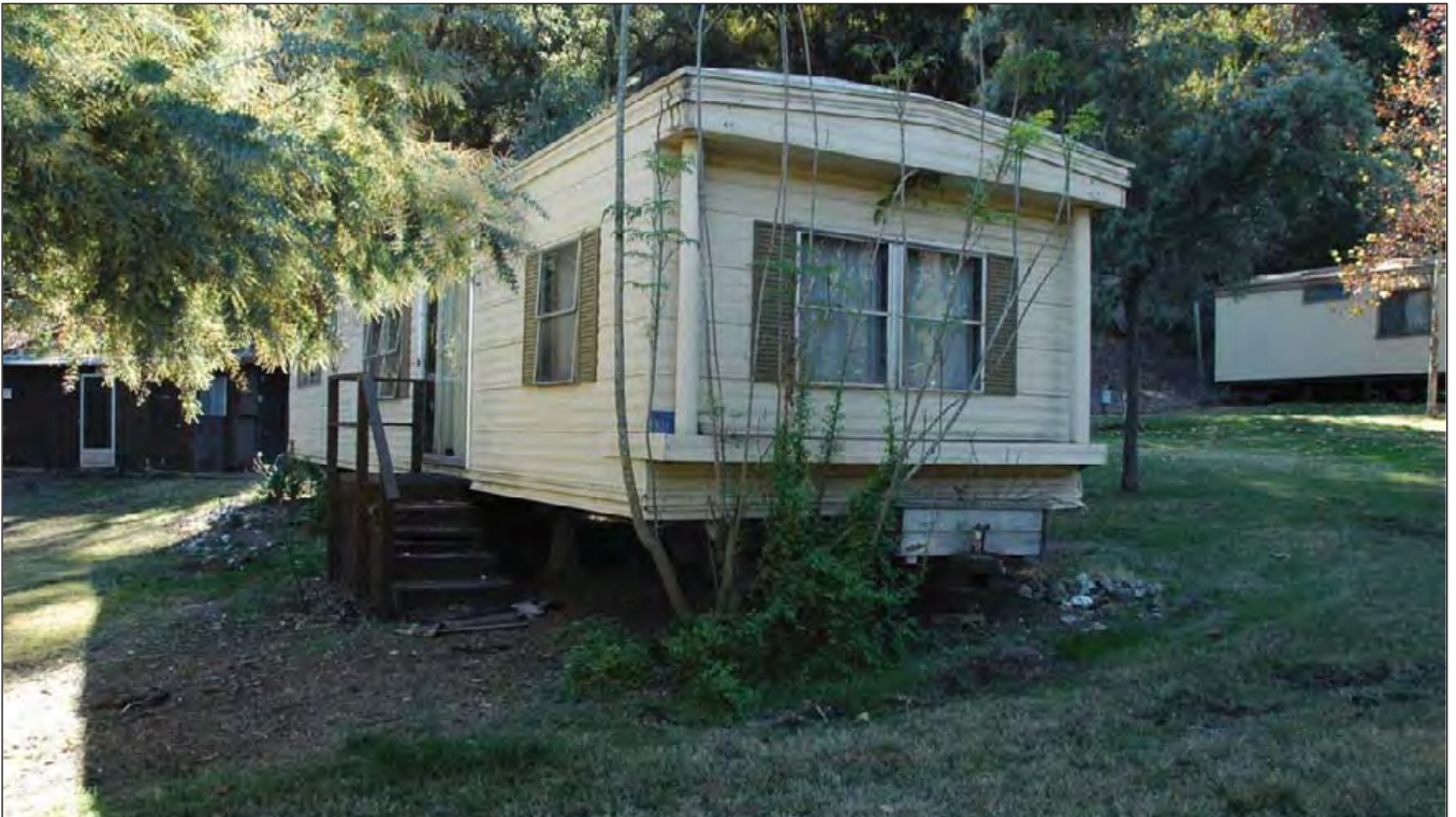
Photo: View of one of the existing mobile homes located in the southern portion of the Project Site.
