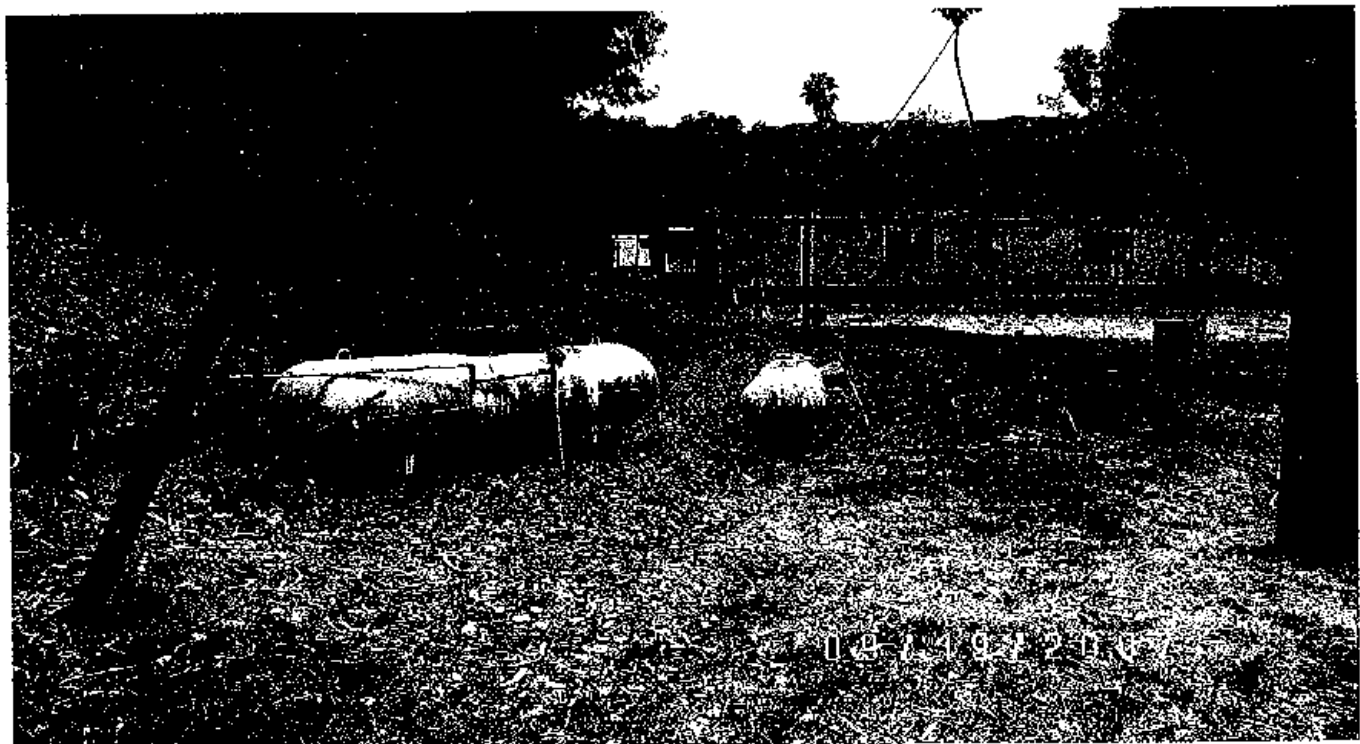
10. VIEW OF PROPANE TANKS AT TRAILER HOOK-UP LOCATIONS.
