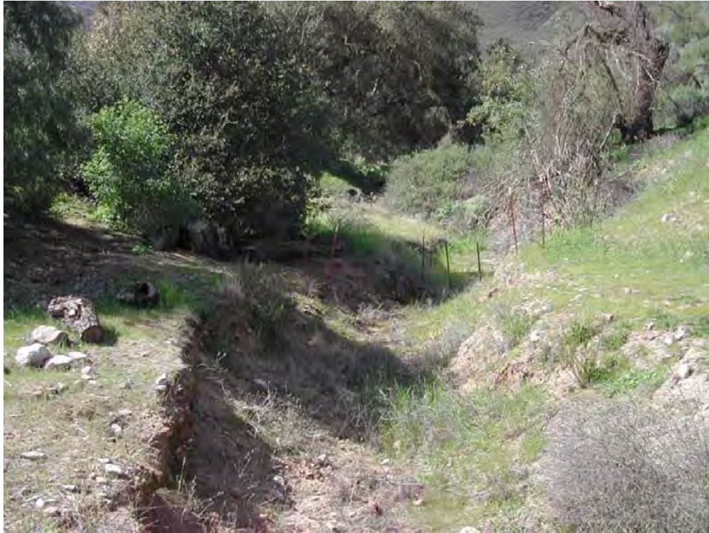
Photo 7: Main drainage channel looking upstream, just upstream from Photo 8
