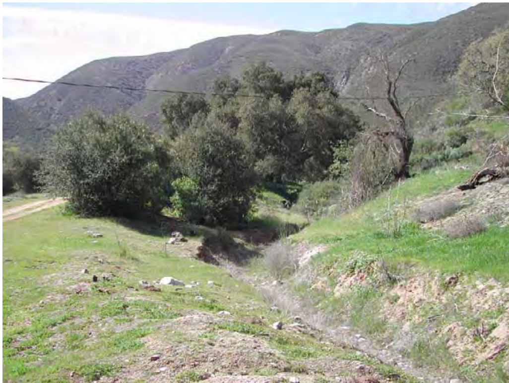
Photo 6: Main drainage channel looking upstream, downstream of Photo 5 and downstream of Photo 7
