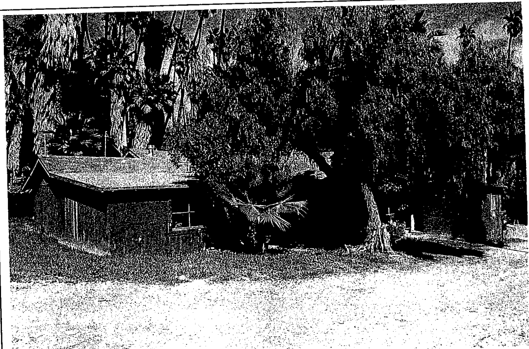
Photo 20: View of the Lodge from the southeast.
