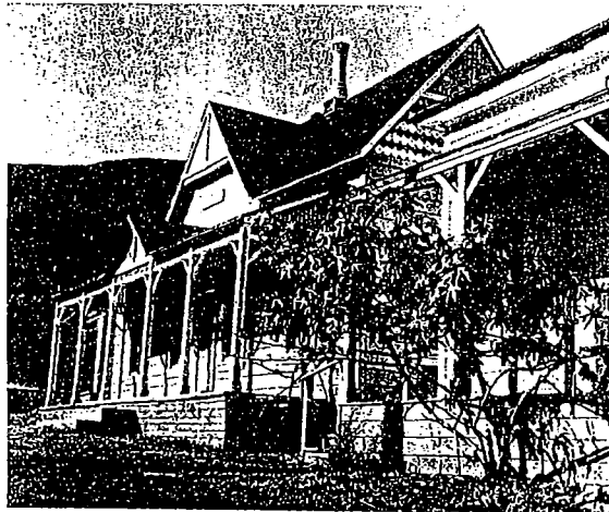
VICTORIAN COTTAGES are in the process of restoration which is supervised by the springs manager, Mrs. Jacqueline Revis. Handling the actual reconstruction is Ole Hellekson who spends much of his time at the resort turning back the clock with his restoration work. Many of these cottages are now as they were at the turn of the century before two destructive fires razed the property in 1928 and again in 1934.
