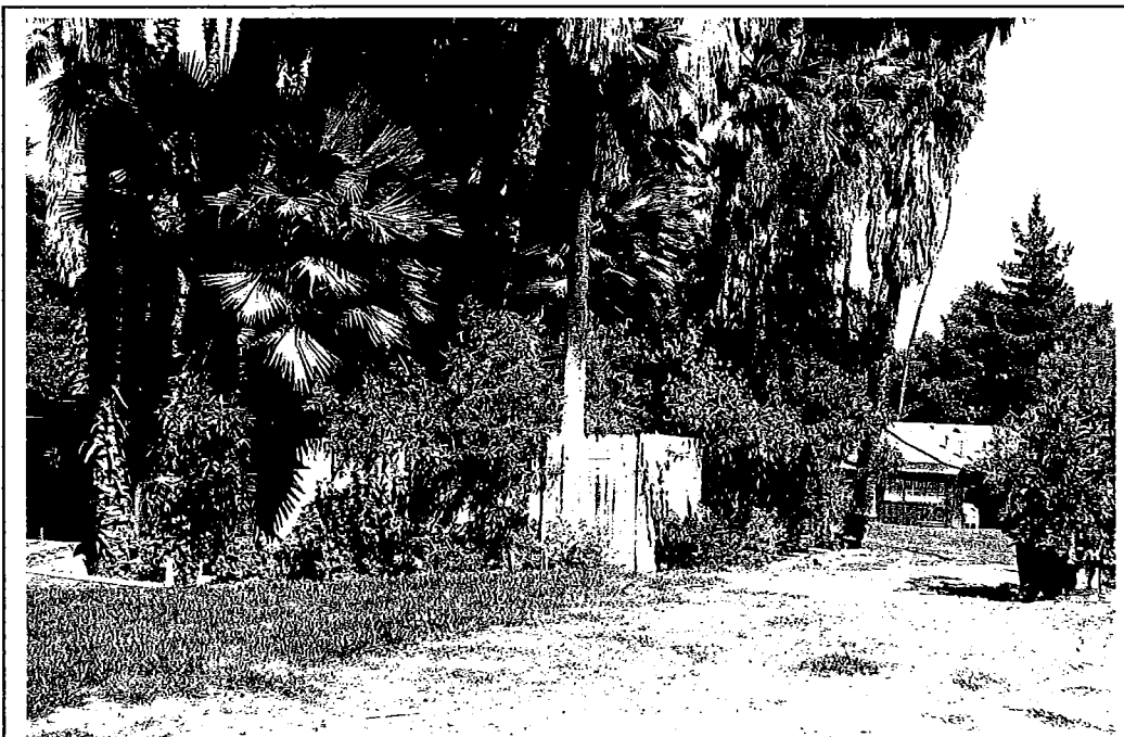
Photo 6: View of the fence enclosure around Hot Bath building and dressing room.
