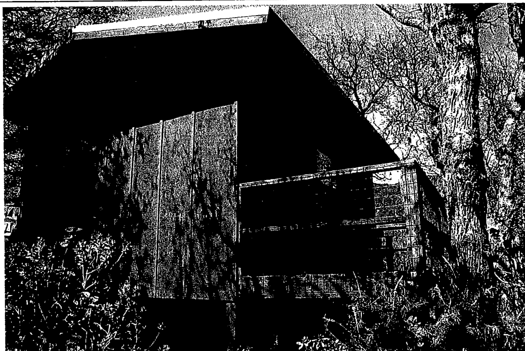
Photo 48: Detail of balcony of Hillside Cabin #13.
