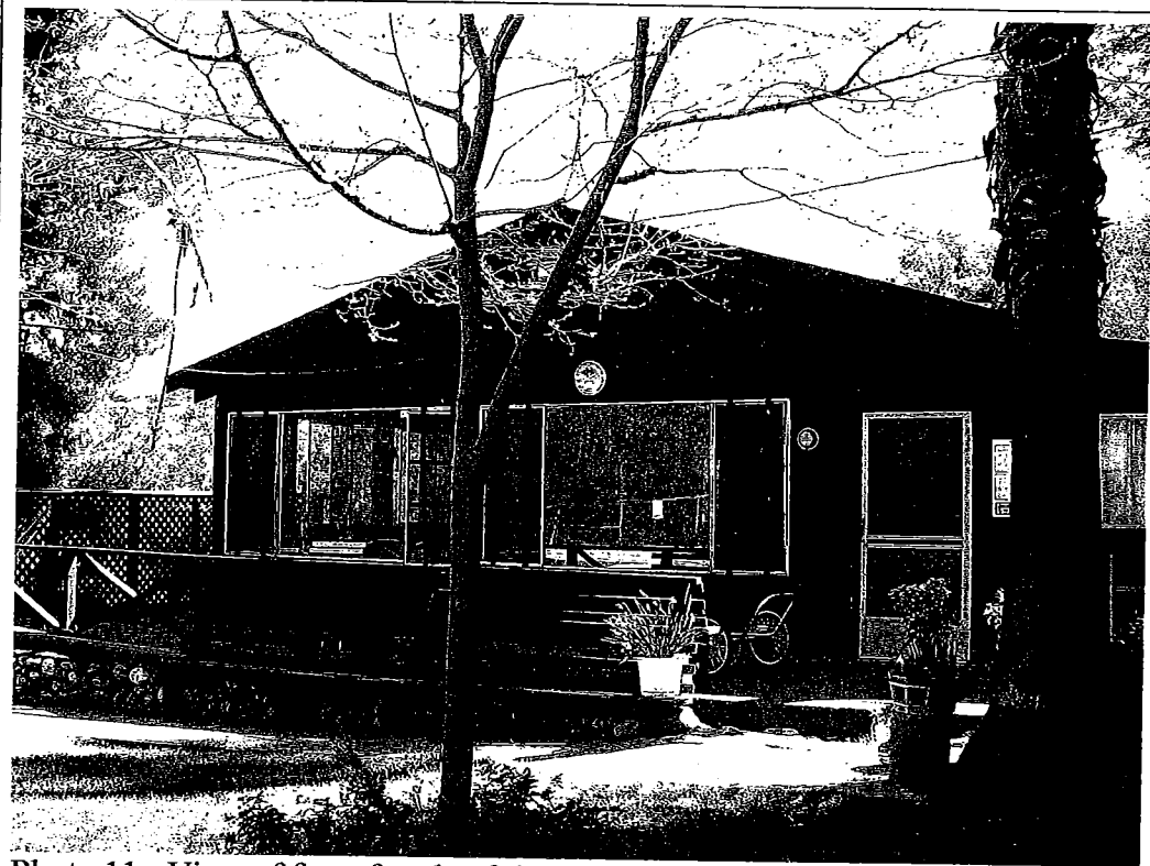
Photo 11: View of front façade of the Recreation Room.
