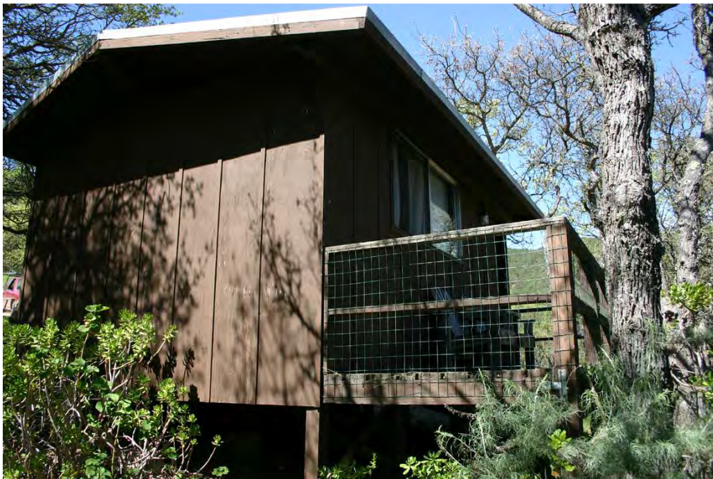
Photo 48: Detail of balcony of Hillside Cabin #13.
