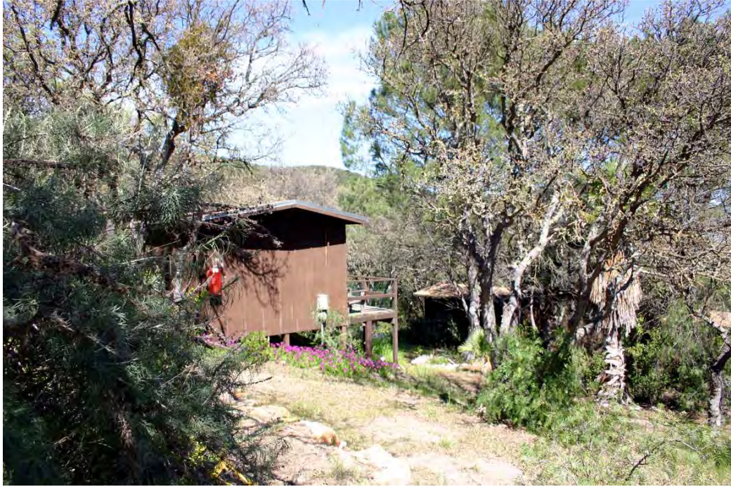
Photo 45: View of the side façade of Hillside Cabin #13.
