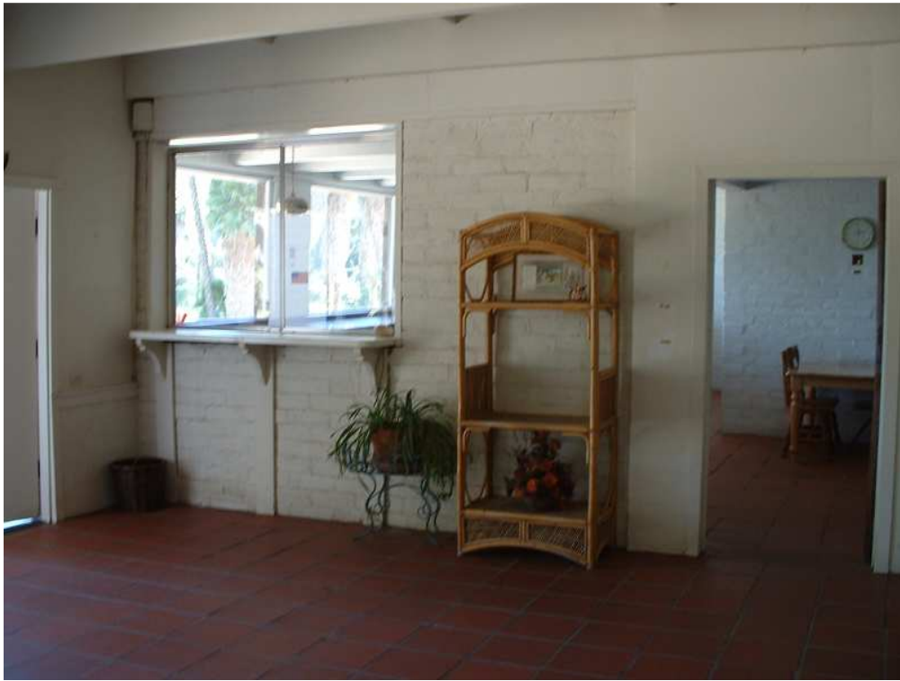
Photo 27: Detail of brick interior wall separating living room from snack bar.
