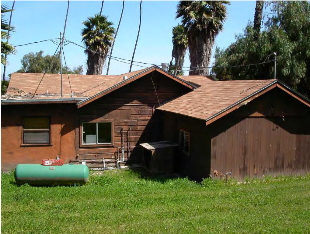
Photo 21: View of the rear façade of the Lodge. Note gabled roof.
