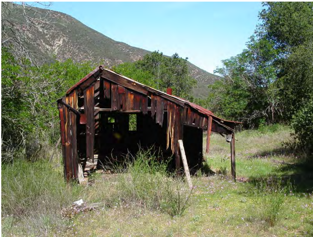
Photo 54: View of gable end façade of the "Miner's Shack".
