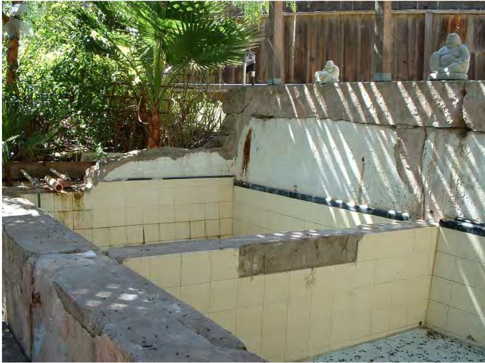
Photo 15: View of the interior of the Old Baths. Note original ceramic tiles.
