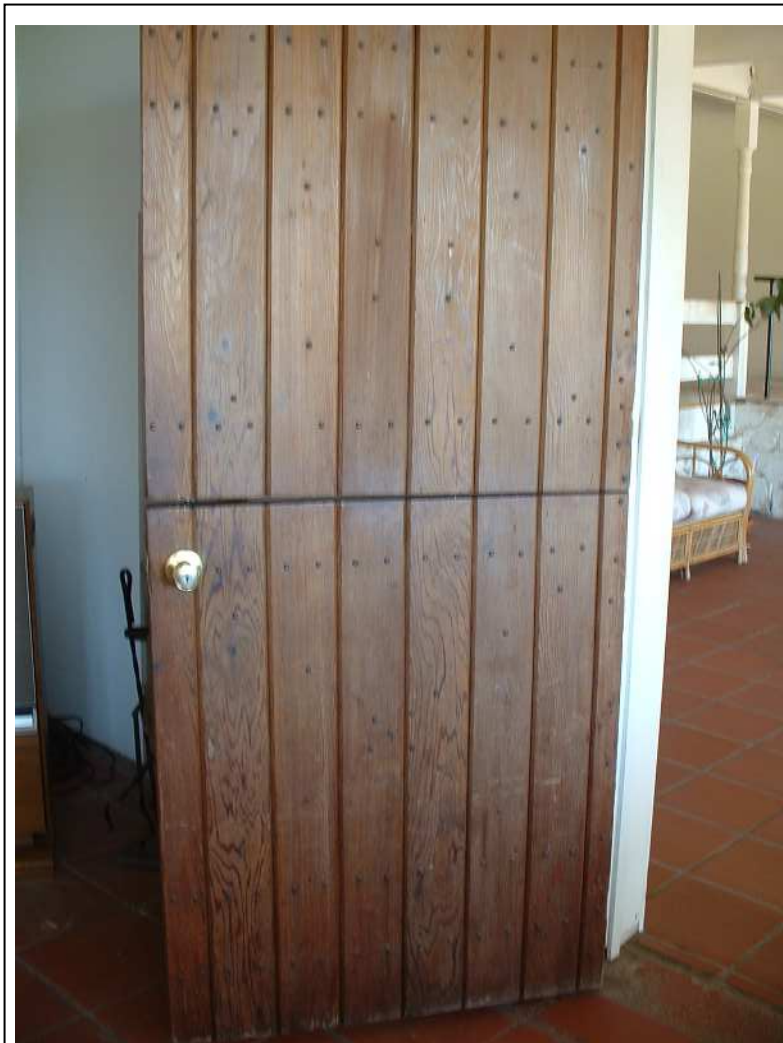
Photo 30: Detail of plank door of snackbar.
