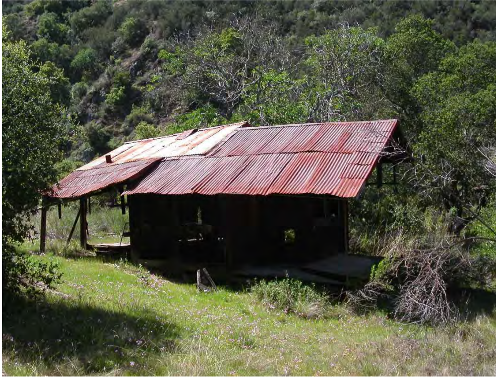
Photo 53: View of the "Miner's Shack." Note red metal sheeting on roof.
