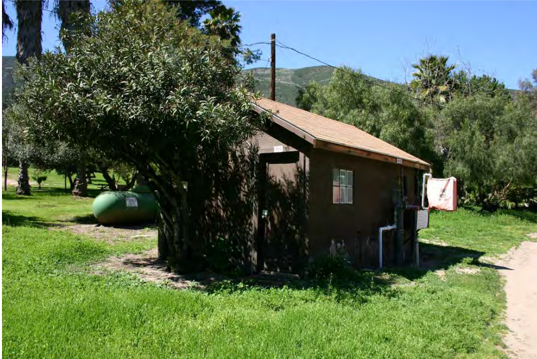
Photo 37: View of bathrooms presently extant in Palm Court area.
