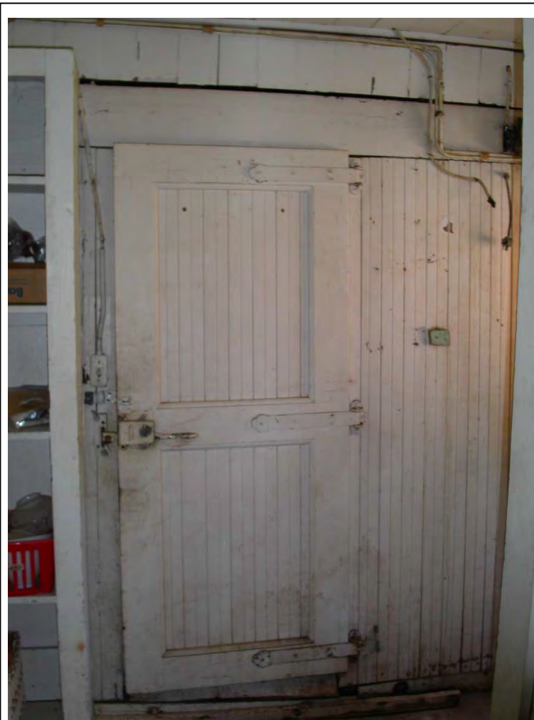
Photo 34: Detail of door to historic walk-in refrigerator off of kitchen.
