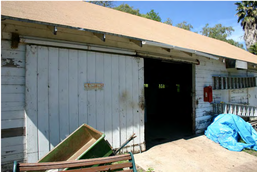
Photo 39: View of vehicular entrance to workshop.
