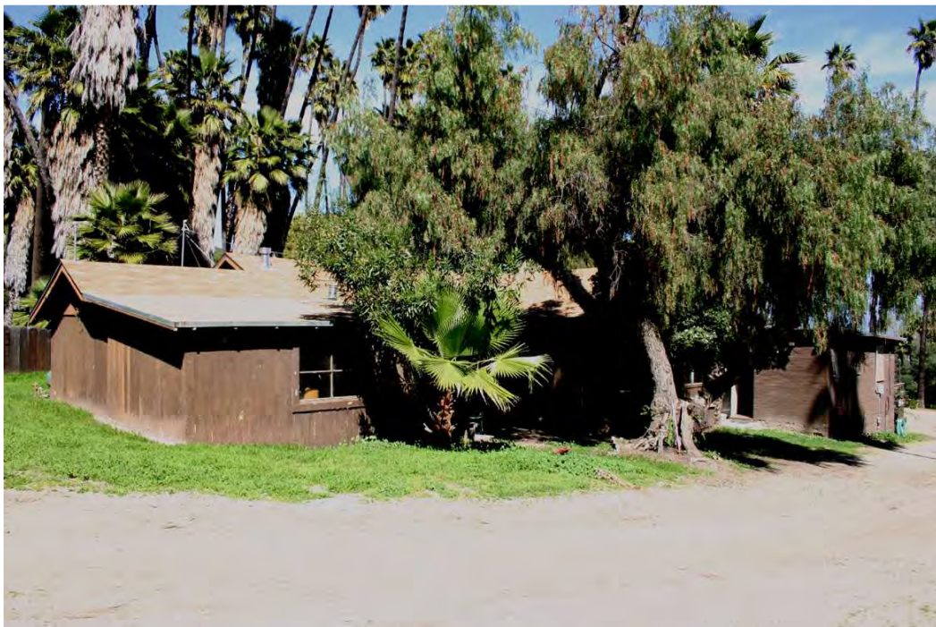
Photo 20: View of the Lodge from the southeast.
