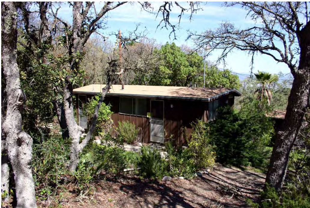
Photo 52: Restroom and shower building in the Hillside Cabins area.
