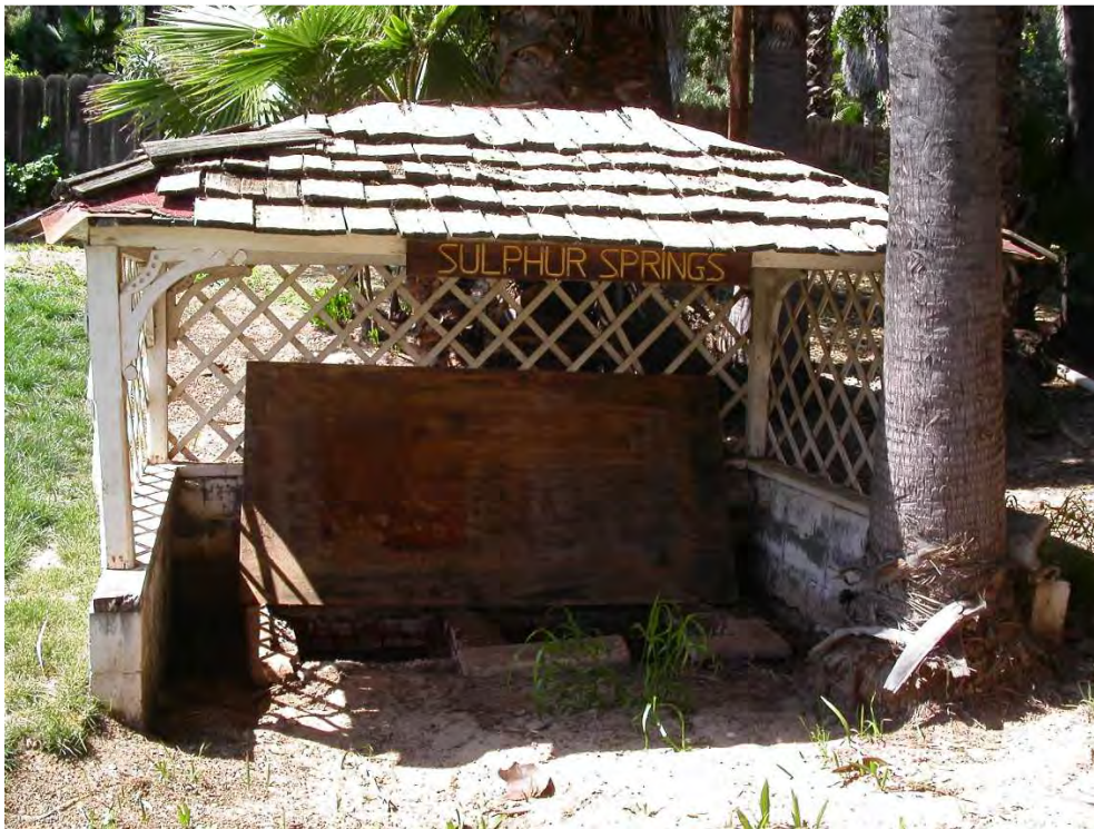
Photo 5: View of canopy shelter over the Sulphur Springs.
