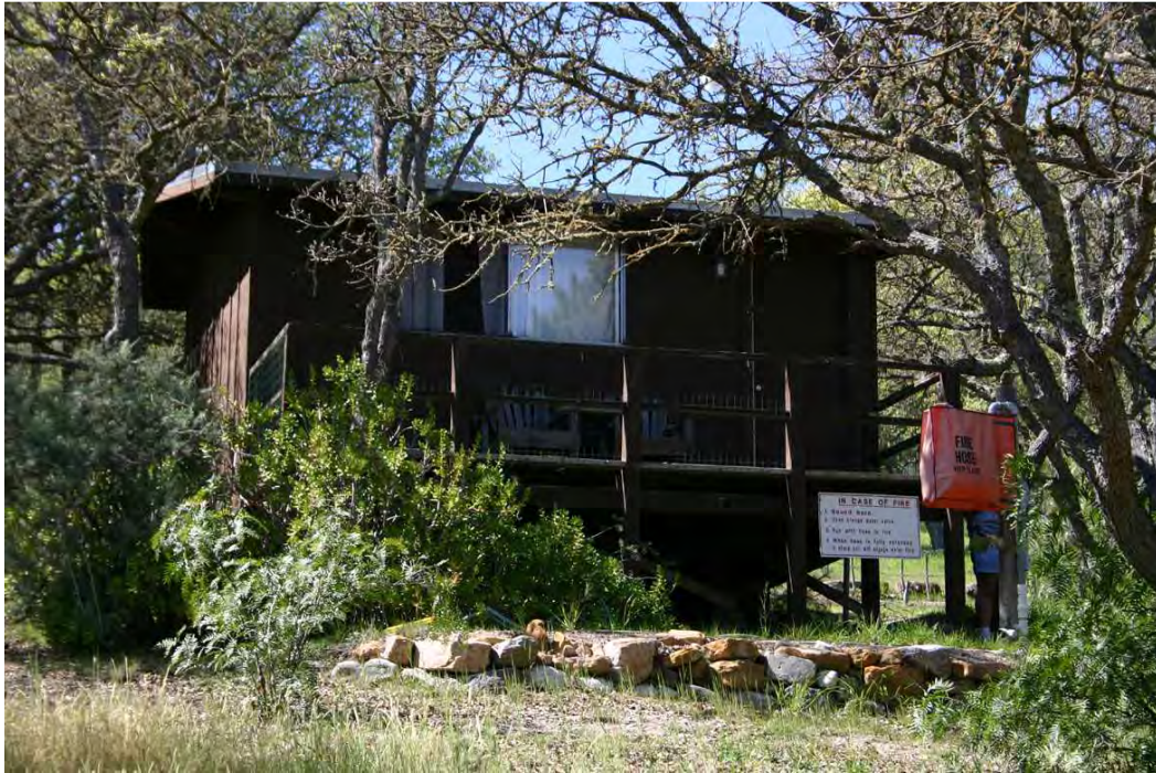
Photo 49: View of rear façade of Hillside Cabin #13.
