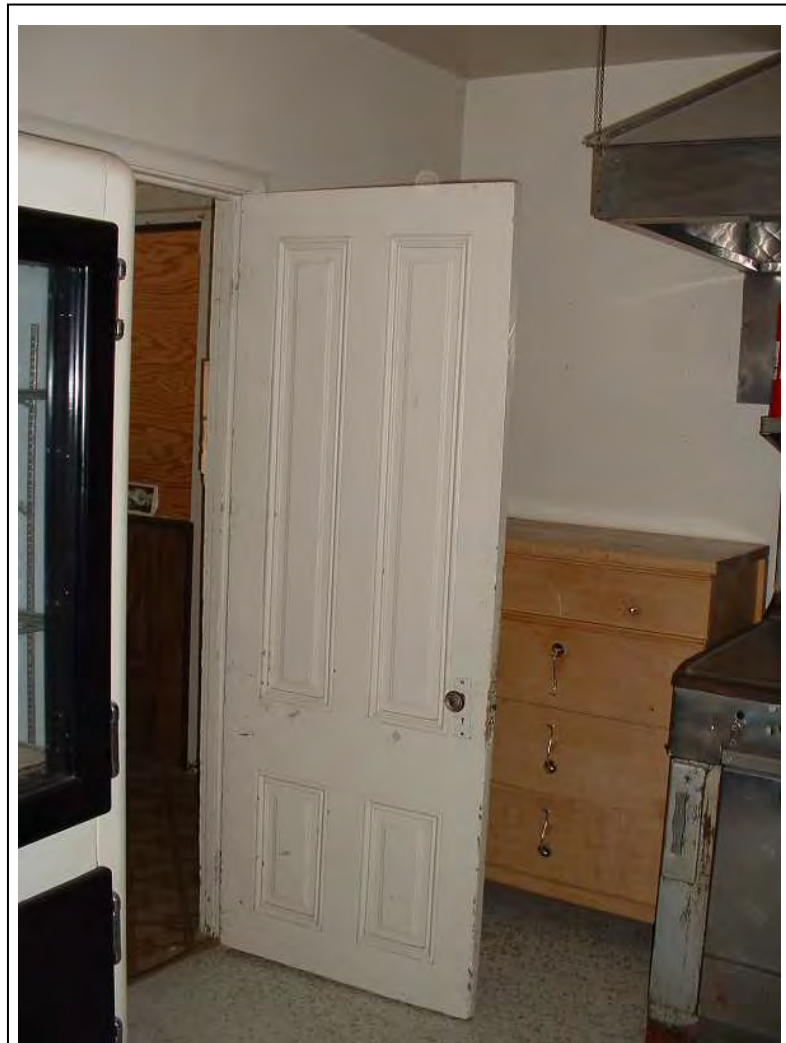
Photo 33: Detail of panel door into kitchen.
