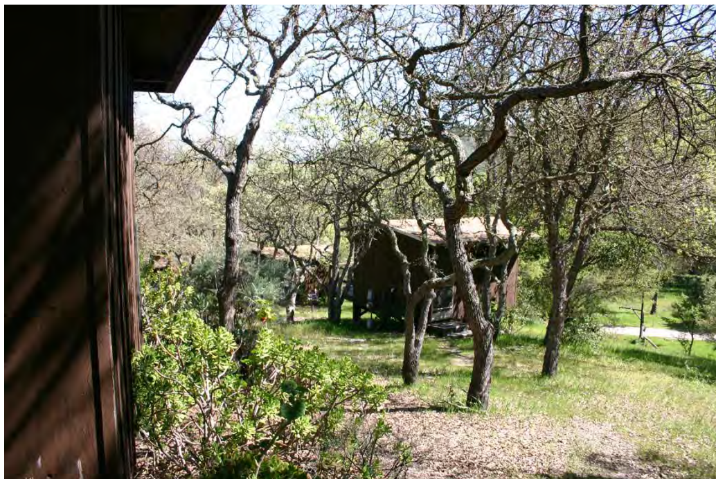
Photo 44: View of Hillside Cabins.
