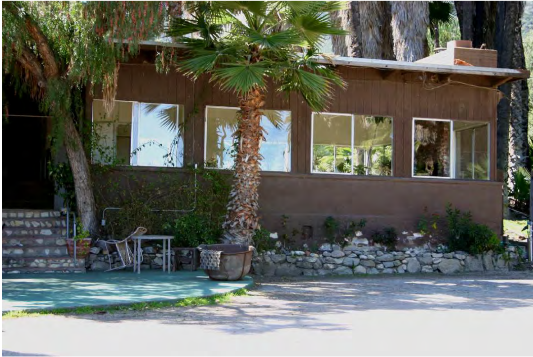
Photo 17: Detail of northern half of front façade of the Lodge.
