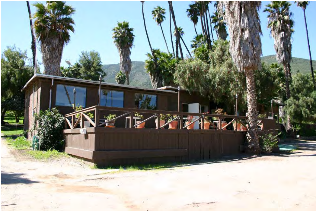
Photo 19: View of deck and southern half of the front façade of the Lodge.
