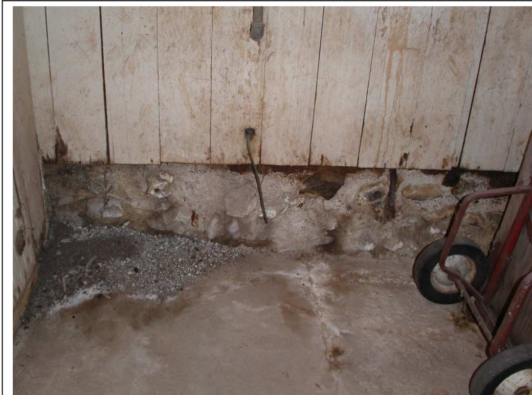
Photo 36: Detail of "soil-cement" foundation in rear of lodge.
