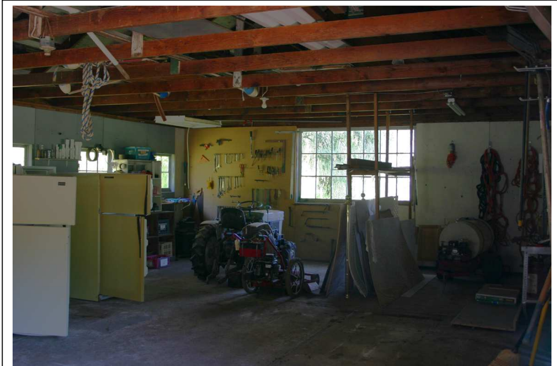
Photo 41: View of interior of the workshop.
