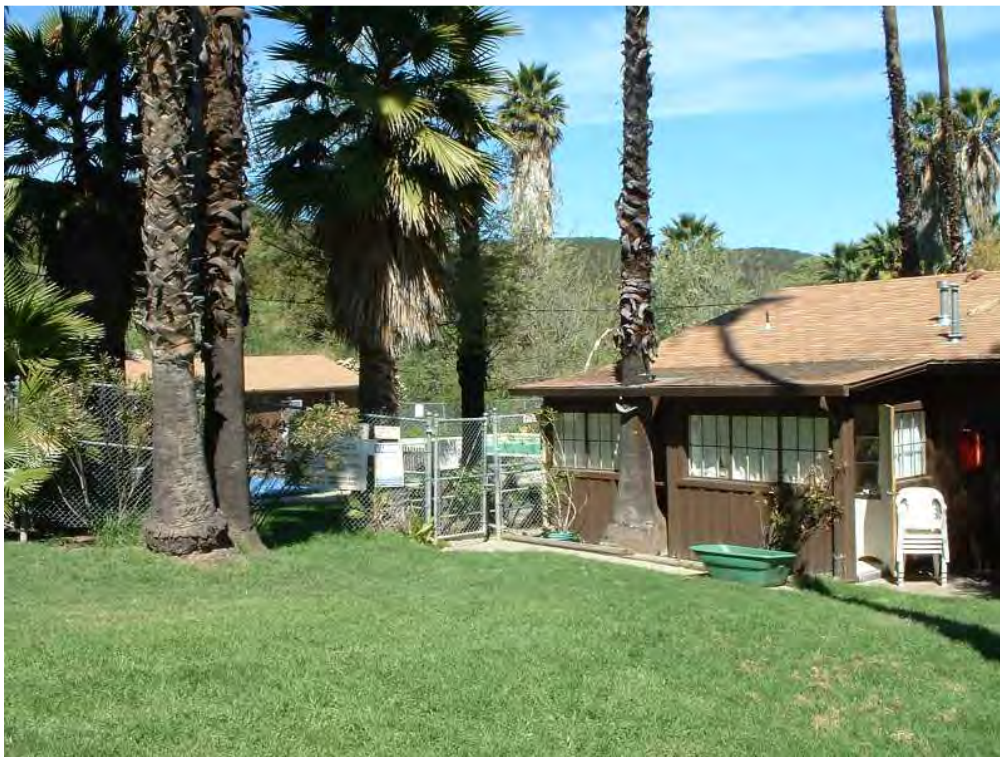
Photo 8: View of the Recreation Room and adjoining lawn.
