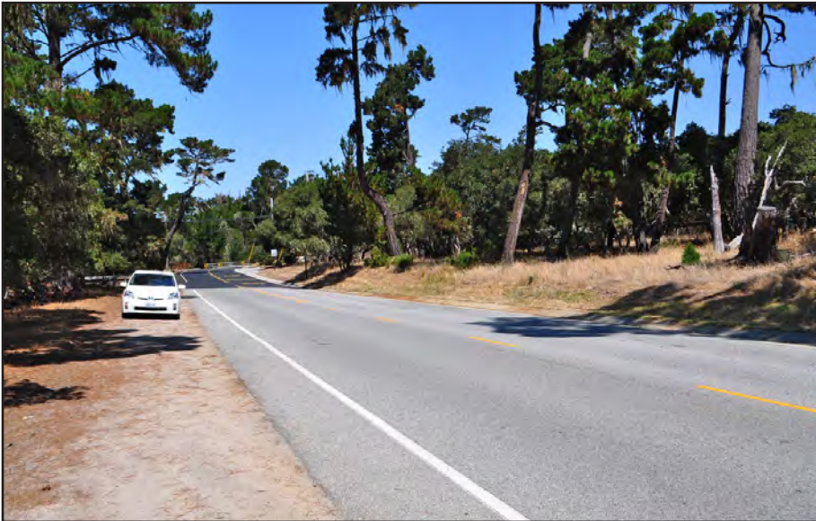
7. Looking north from SFB Morse Drive toward the roadway curve and forest buffer area.
