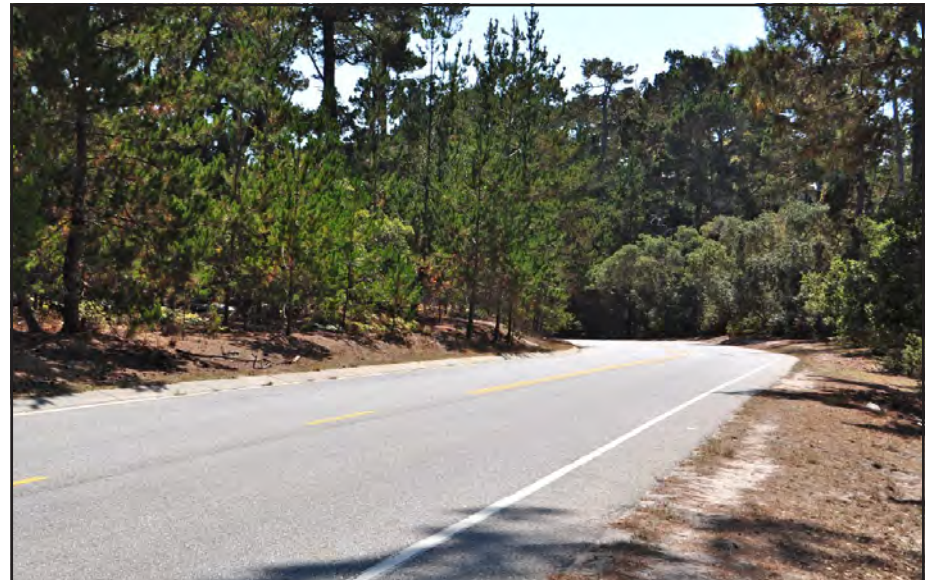
8. Looking south from SFB Morse Drive toward the roadway curve and forest buffer area.
