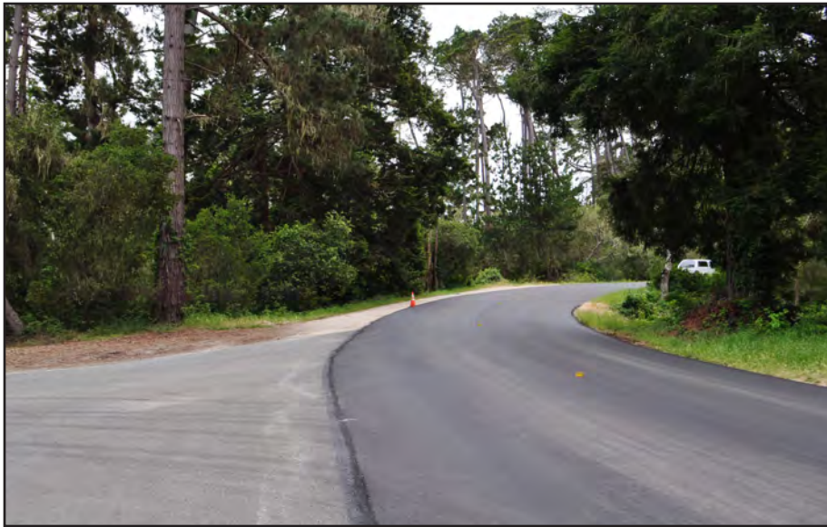
24. Looking southwest from Stevenson Drive toward Area K.
