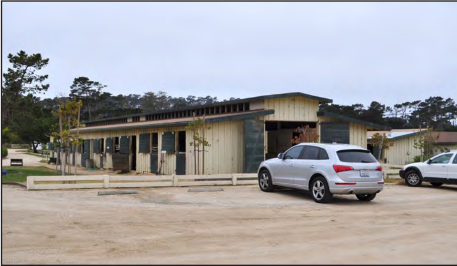
11. Looking west from the Equestrian Center parking lot toward the stables.
