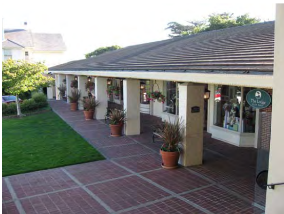
West wing of the Lodge Annex. (Page & Turnbull, November 2012)
