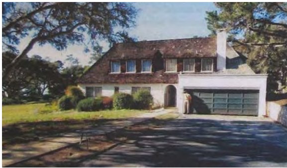
“Pinewood Edge,” a French Eclectic house built in 1924 at 3414 17-Mile Drive and designed by architect Houghton Sawyer. It was demolished ca. 2011. (LSA Associates, 31 August 2009, DPR 523 A form photo on file with the Monterey County Planning Department)
