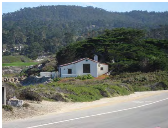
Monterey Peninsula Country Club bath house, designed by Clarence Tantau. (Page & Turnbull, November 2012)
