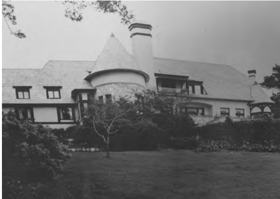
Peter Stolich house, 3950 Ronda Road, circa 1953. (Courtesy Pebble Beach Company Lagorio Archives)
