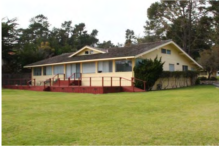
The “Canary Cottage,” constructed circa 1914. (Page & Turnbull, March 2013)
