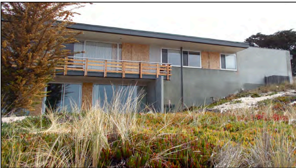
Photo 6. Western elevation, southern half. [1-31-2014]
