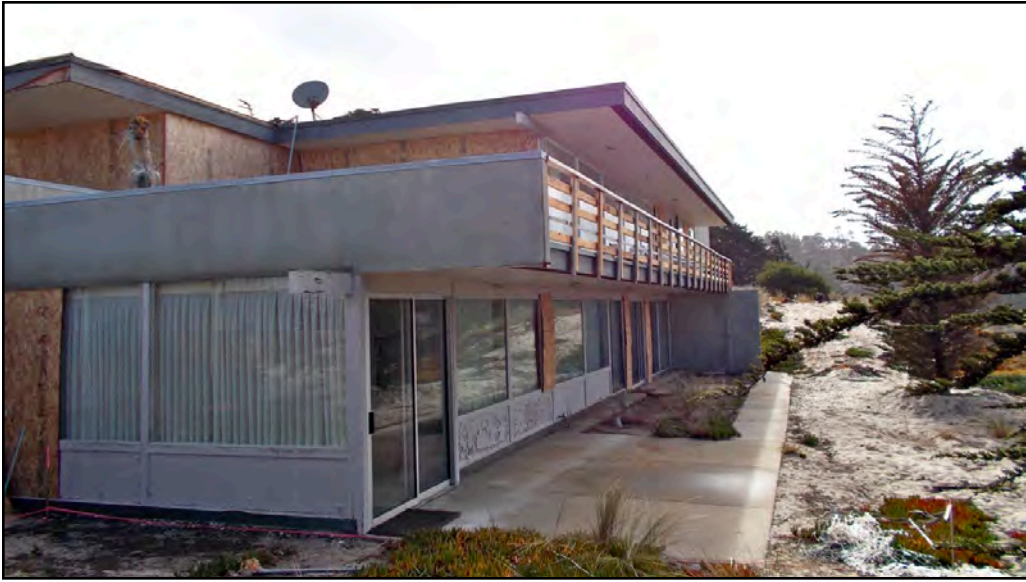
Photo 4. Northern and western elevations. [1-31-2014]
