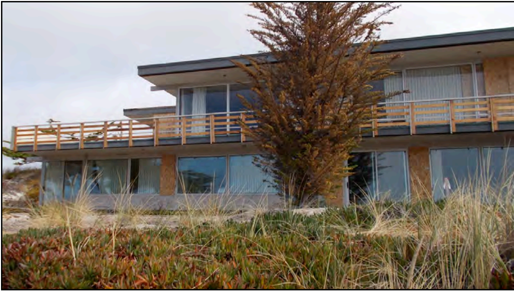
Photo 5. Western elevation, northern half. [1-31-2014]
