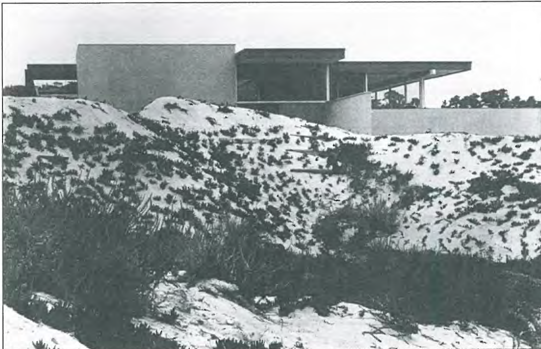
Figure A. Looking south at north elevation.
