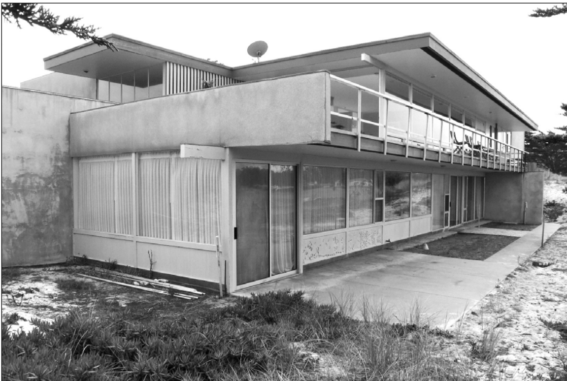
Figure 2. Looking southeast at north and west sides, 5 October 2010.
