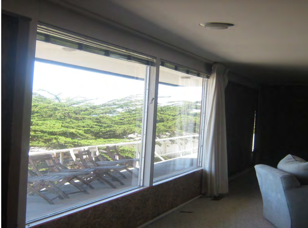
Picture 4 - Replacement Windows Remaining - Living Room
