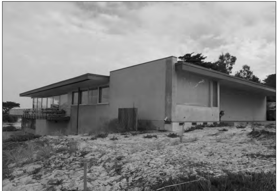
Figure 2. Looking northeast at west and south elevations, 10/5/10.
