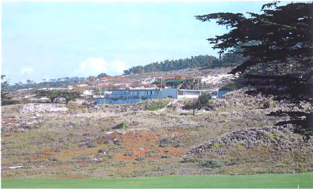
IMAGE 13 Cypress Point Club: From the eastern edge of the golf course looking northeast, the house is still silhouetted by the dune hillside and existing trees.
