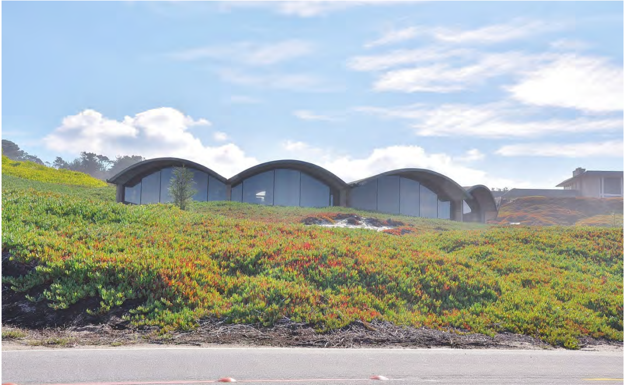
IMAGE 21 Adjacent Homes: This well-known architectural home directly on 17 Mile Drive offers no ridgeline protection at all.
