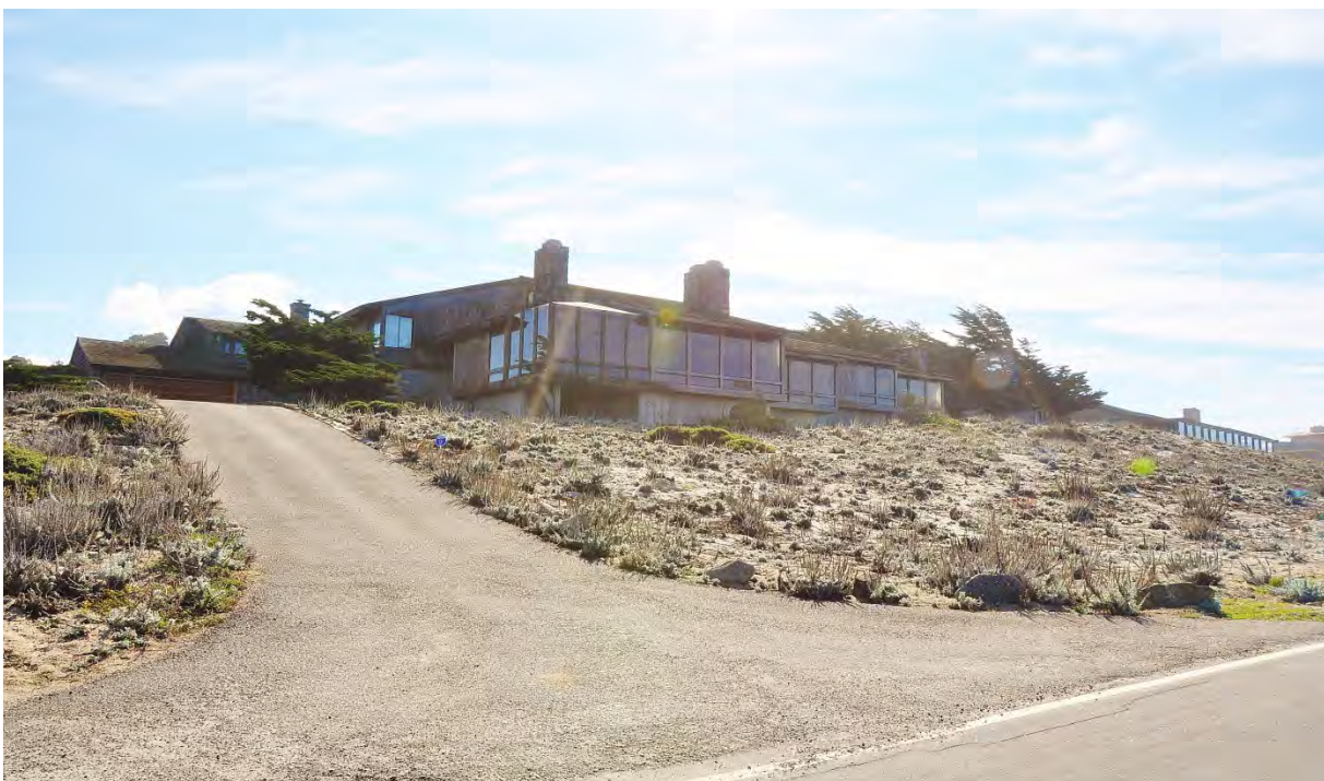
IMAGE 22 Adjacent Homes: Another home directly on 17 Mile Drive.
