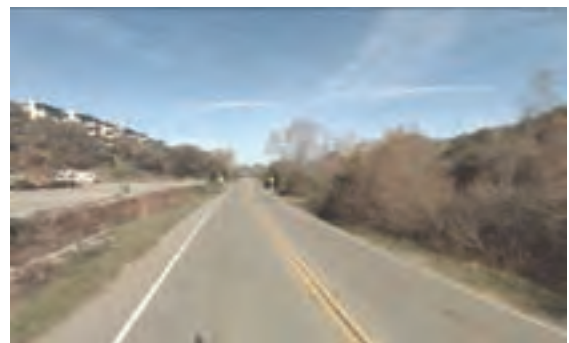
The shoulders in many places along Canyon del Rey are narrow.
