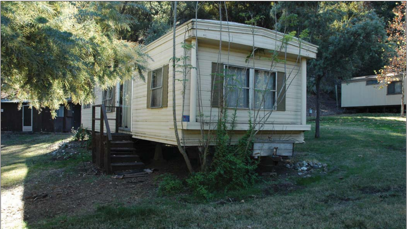
Photo: View of one of the existing mobile homes located in the southern portion of the Project Site.
