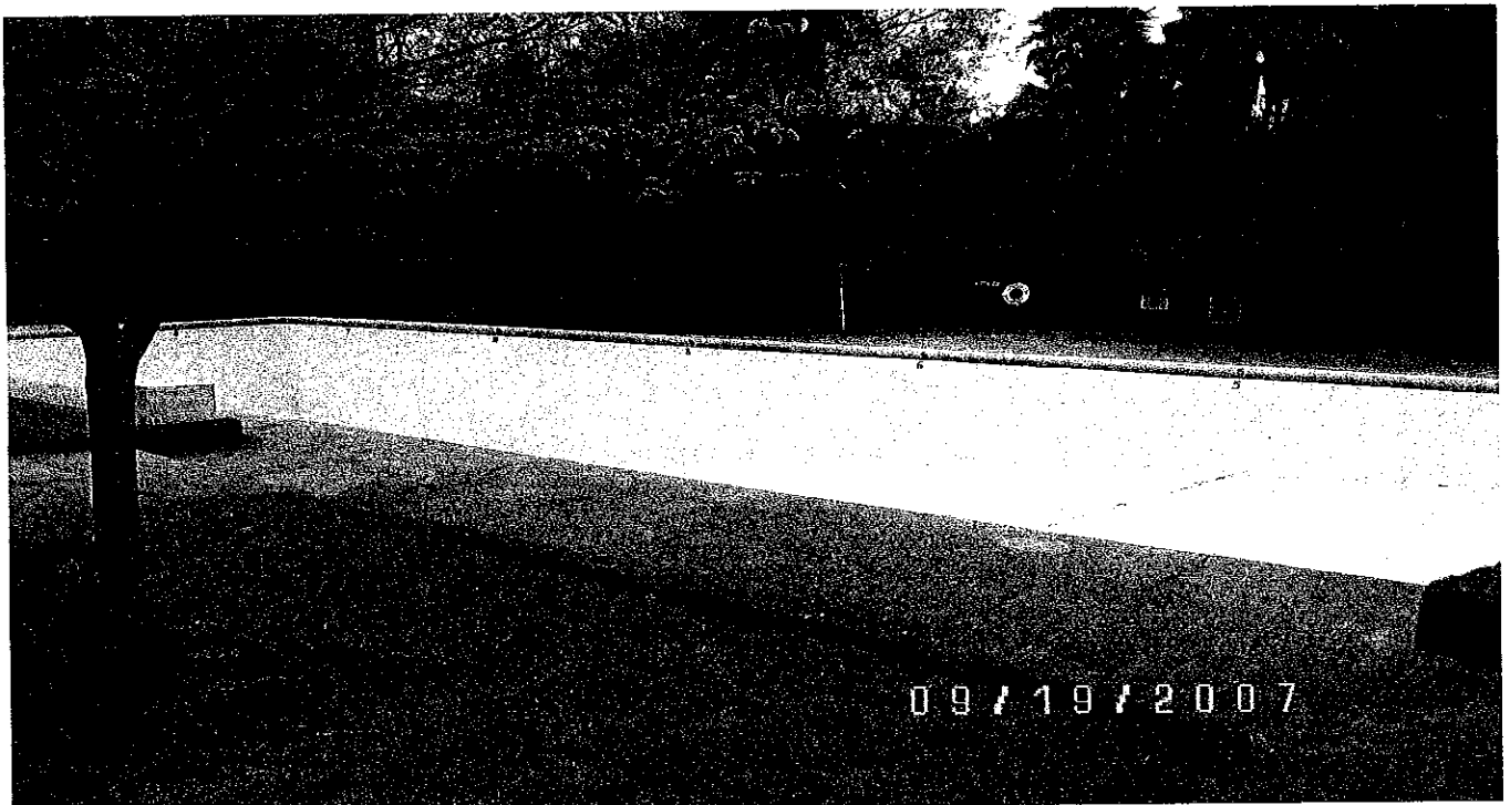
8. SECOND POOL SHOWING CONSTRUCTION.
