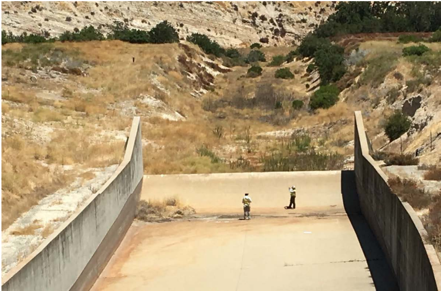
Flip Bucket and Exit Channel
