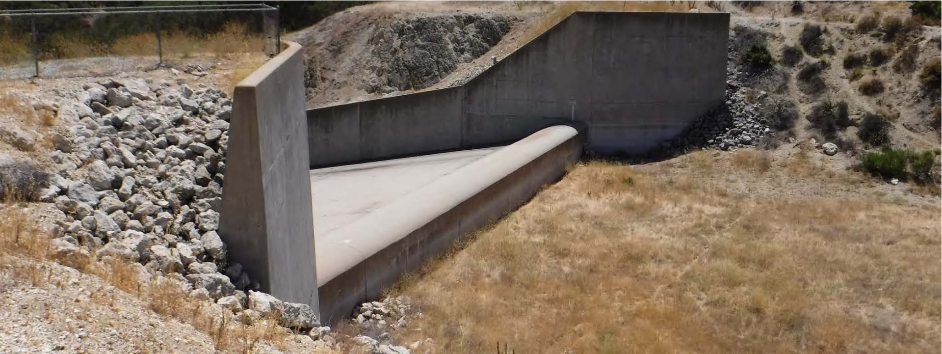
Concrete Ogee Weir
