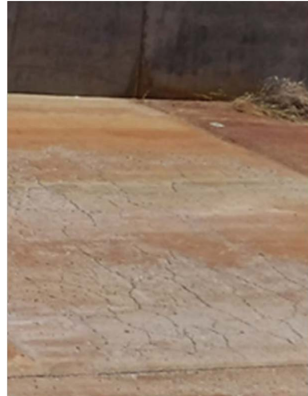
Example Concrete Condition
