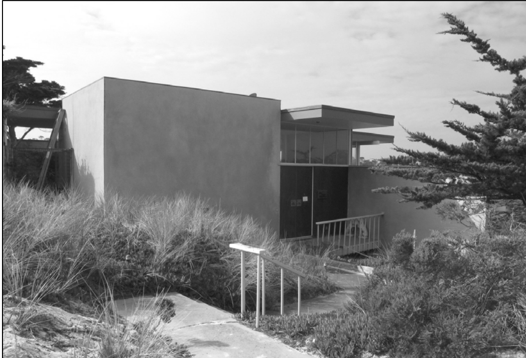
Figure 4.3-6. North elevation, looking southwest.
