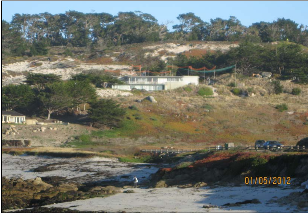
Figure 4.3-2. West elevation, looking east from 17-Mile Drive.
