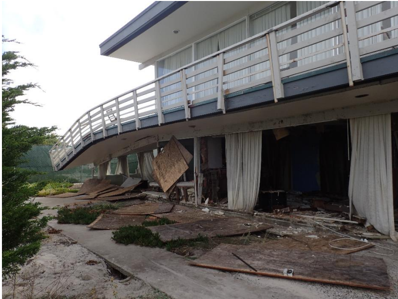
Photo 5 SWCA photo looking north along the building's west face.
