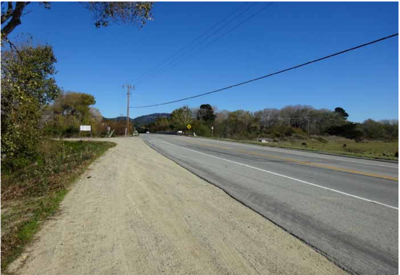
1. View of central part of Subject Property Highway One area, looking north.
