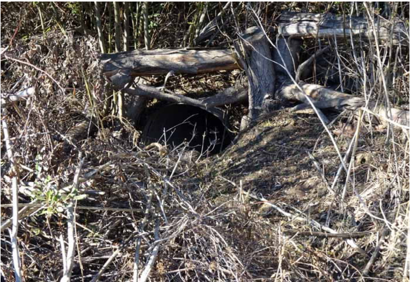
8. View of drain pipe that runs beneath the east part of the property.
