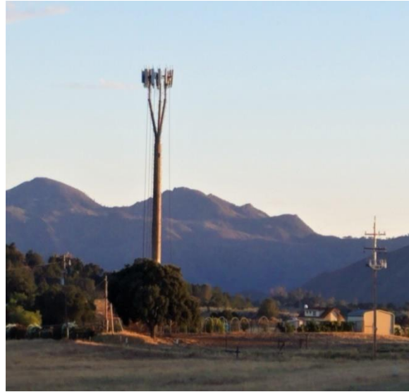
Tuesday, August 6 th , 2019 Tower Construction
