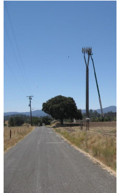
HESPERIA ROAD -- CELL TOWER CONSTRUCTION
