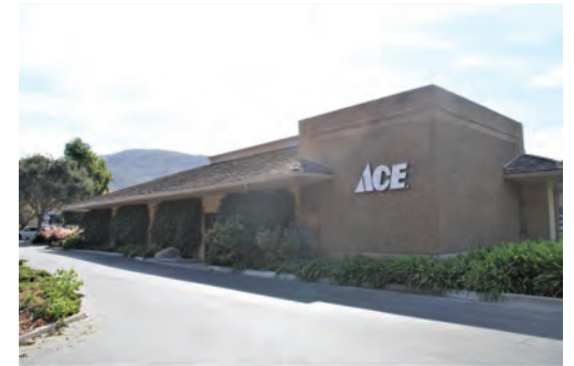
④ Building D - Ace Hardware
